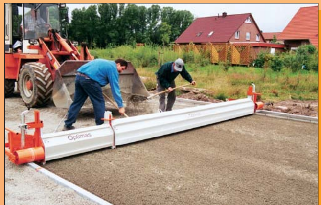
The rolling units are individually height-adjustable so that existing curbs or gutters and the Optimas rails can be flexibly combined for screeding.
