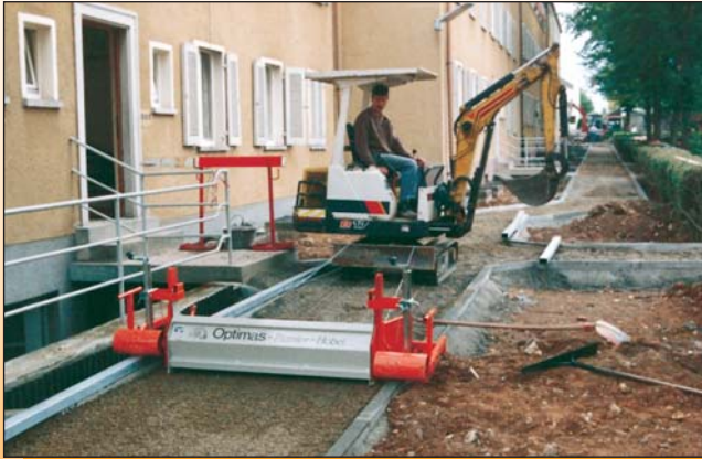
Screeding of a 1.2 m wide footpath.
